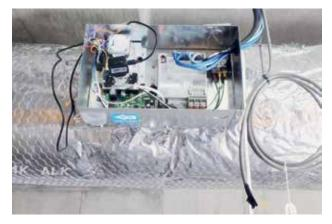
A variable air volume unit being monitored for signal exchanges and the angle of the opening control valve. Source: EBC Working Group on HVAC Energy Calculation Methodologies for Non-residential Buildings the controls. Some calculation methods clearly state that ideal functions of the controls are assumed, while another has adopted a cautious approach in evaluating the components affected by the controls. However, such compensations due to lack of information may be inevitable at present.
