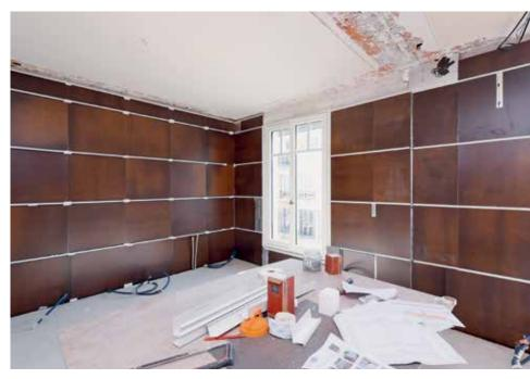
Indoor renovation with vacuum insulation panels finished with a protective layer. Source: SINIAT – CLIMISOL
